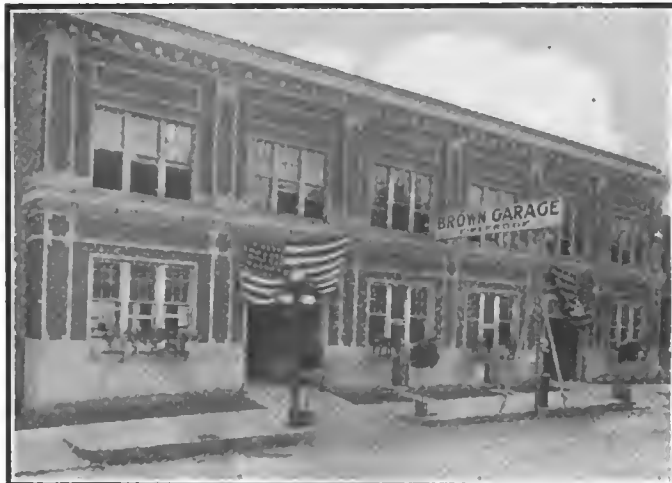
Brown Garage in Des Moines, Ia., which is rendered attractive by means which unfortunately are unusual in garage construction
